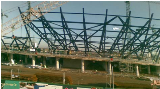
Olympic Stadium under construction
