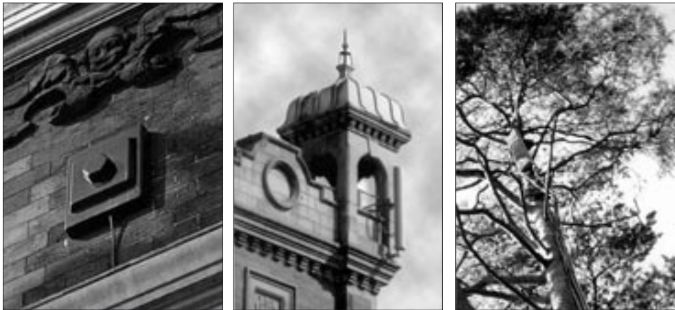
Left: Antenna disguised as an endplate. Centre: Antenna painted to reduce impact. Right: Antenna hidden in a tree.
