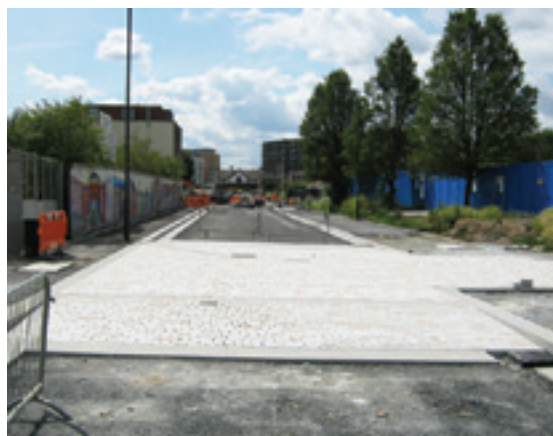
Highways works on Rathbone Street
