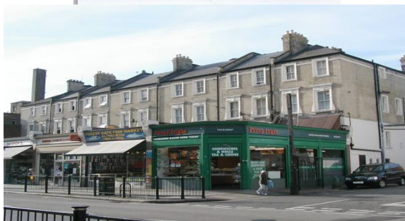
1-13 Woodgrange Road before and after enhancement works.
