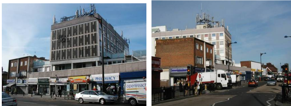
Durning Hall and shops 51-73 Woodgrange Road.
