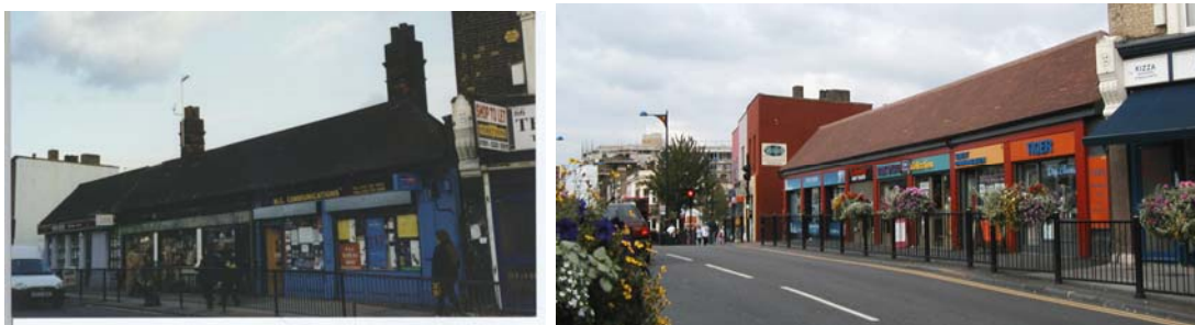
Restoration of the former coal offices on the bridge opposite the station.
