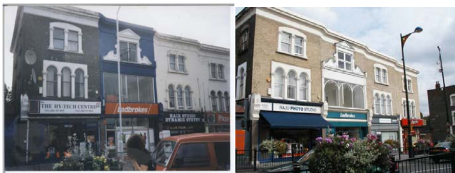
Restoration of Nos: 60 to 68 Woodgrange Road part of the Woodgrange Estate
