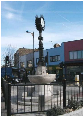
Enhancement works to the Gurney Clock and drinking fountain
