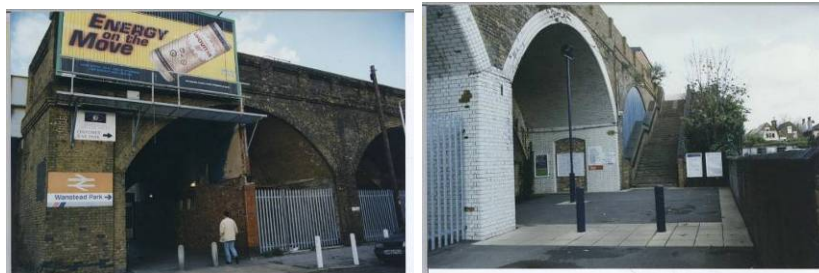
Improvements to access and reuse of arches at Wanstead Park Station
