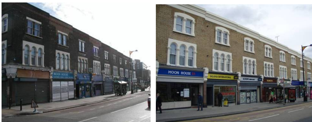
Restoration of 40-58 Woodgrange Road
