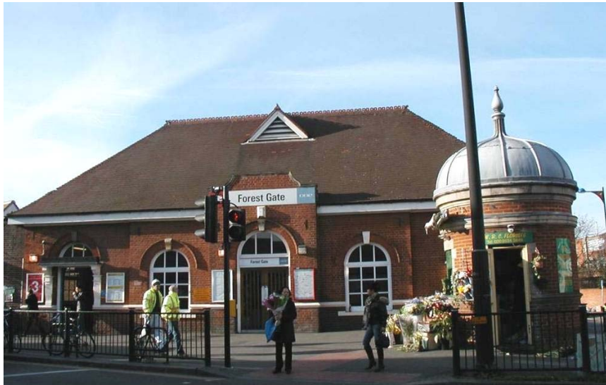
Forest Gate Station facade improvements and kiosk
