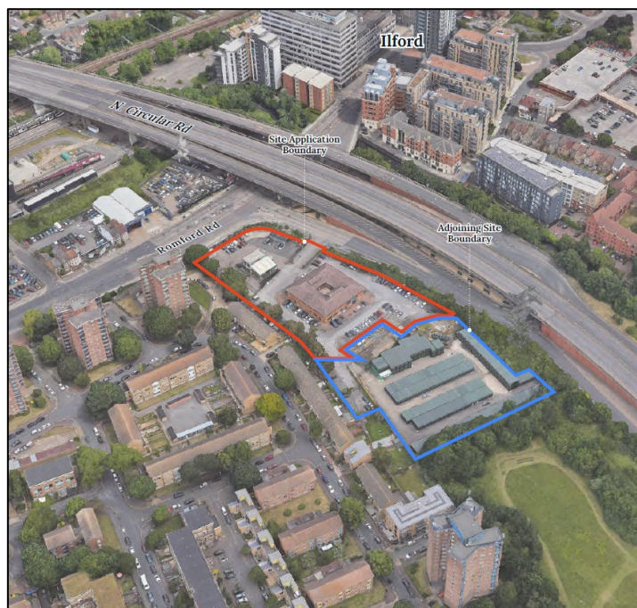
Aerial Photograph – Site Boundary and Adjoining site
