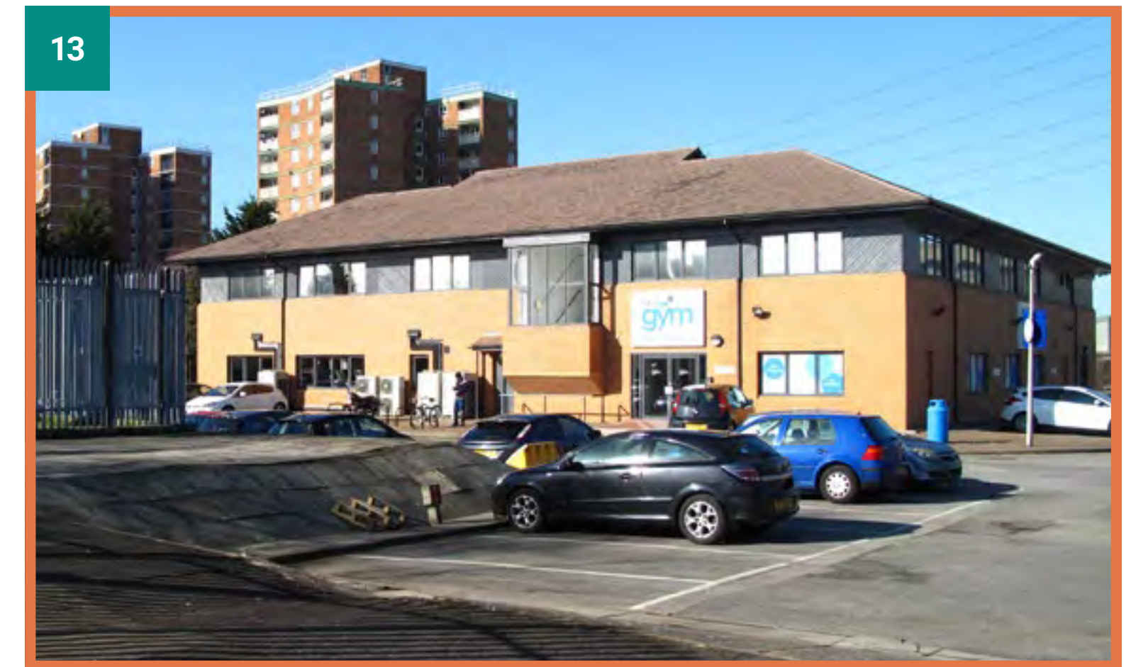
FIGURE 13 THE GYM STREET VIEW
