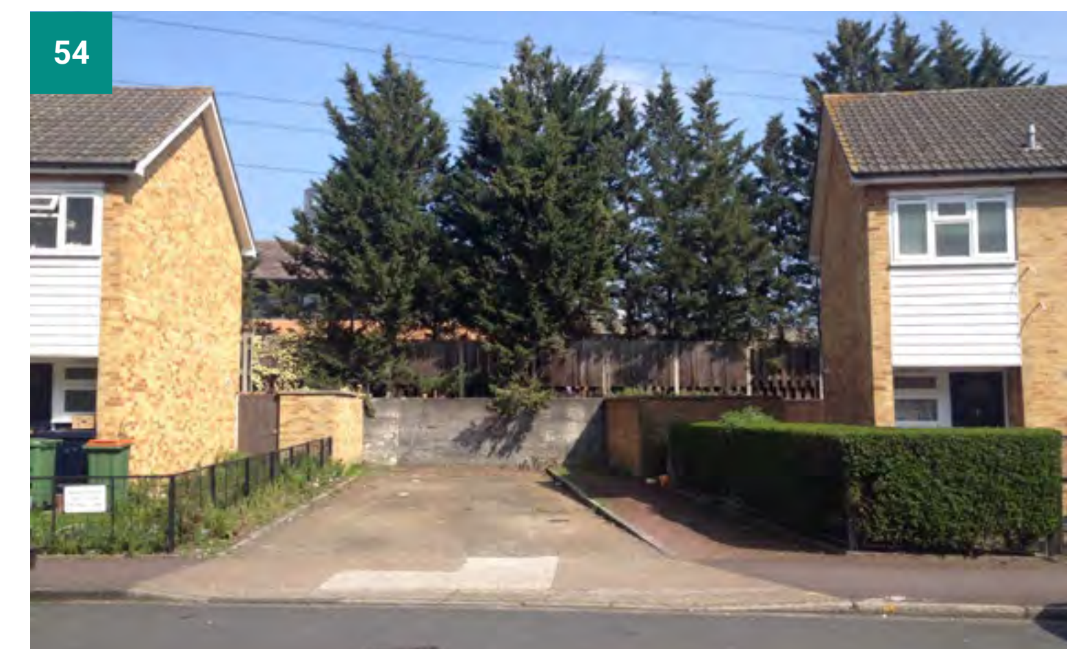
FIGURE 54 SITE PHOTO OF EXISTING RESIDENTIAL ALONG WESTERN BOUNDARY
