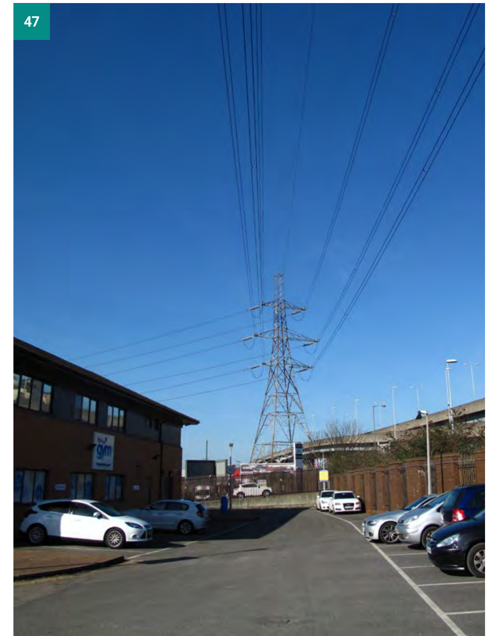
FIGURE 47 SITE PHOTO OF OVERHEAD POWER LINES
