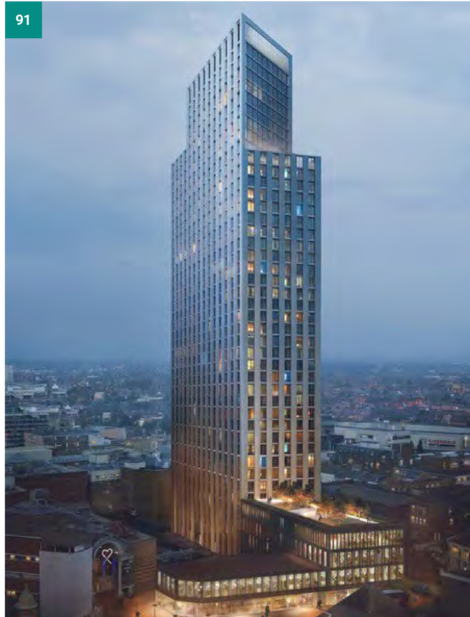
FIGURE 91 ONE STATION ROAD
