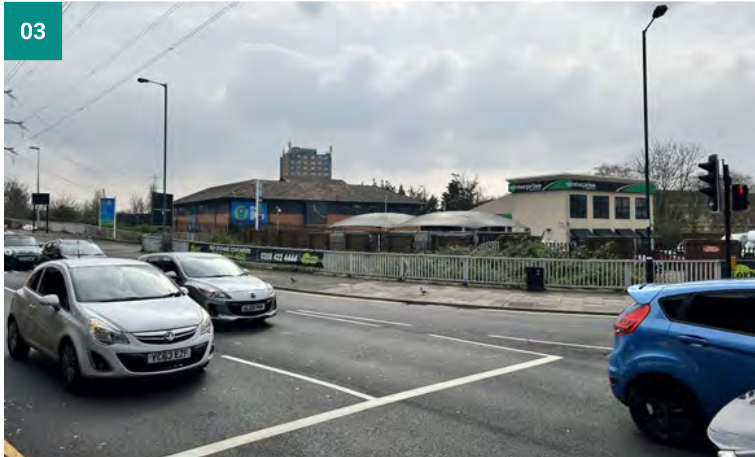
FIGURE 03 SITE PHOTO OF EASTERN BOUNDARY LOOKING SOUTH FROM ROMFORD ROAD
