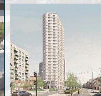
302-312 Stratford High Street 25 storey 240 apartment Aparthotel
