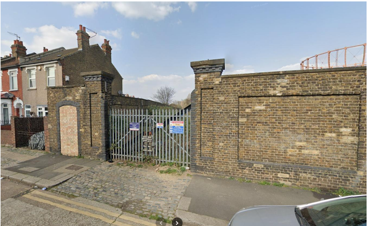
Figure 4 - Photograph taken from south-western corner of the site showing the retained boundary wall, former pedestrian access (bricked up) and National Grid gated access (not currently used) with the gasholder partly-visible.
