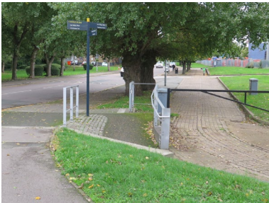
The active travel connection between the towpath at Bow Locks and the Leaway Path, via Twelvvetrees Crescent is unclear and has poor signage. Step-free access to the Leaway route terminates with a gradient which is not compliant for disabled users
