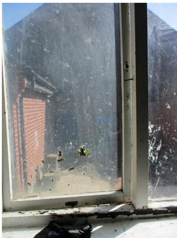
Image above: Ground floor rear kitchen showing casement window with Perspex glazing
