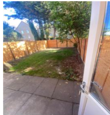
Photo: Back garden with grass, trees and fences cut back and rubbish cleared.
