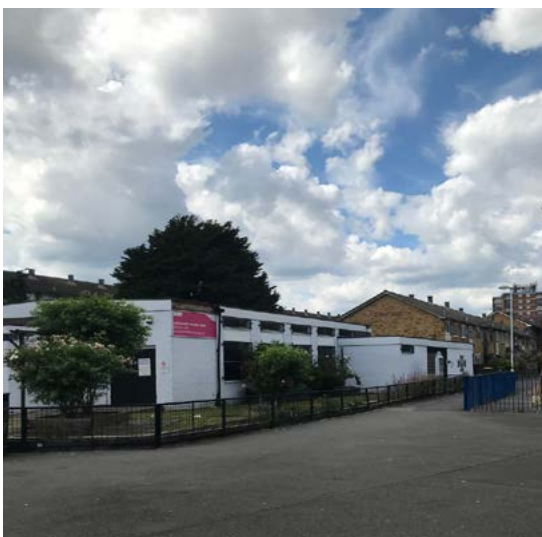
The Jack Cornwell Community Centre is located opposite the shopping parade and hosts a number of activities and support services for both children and adults along with a community café, large hall, and meeting rooms for hire.
