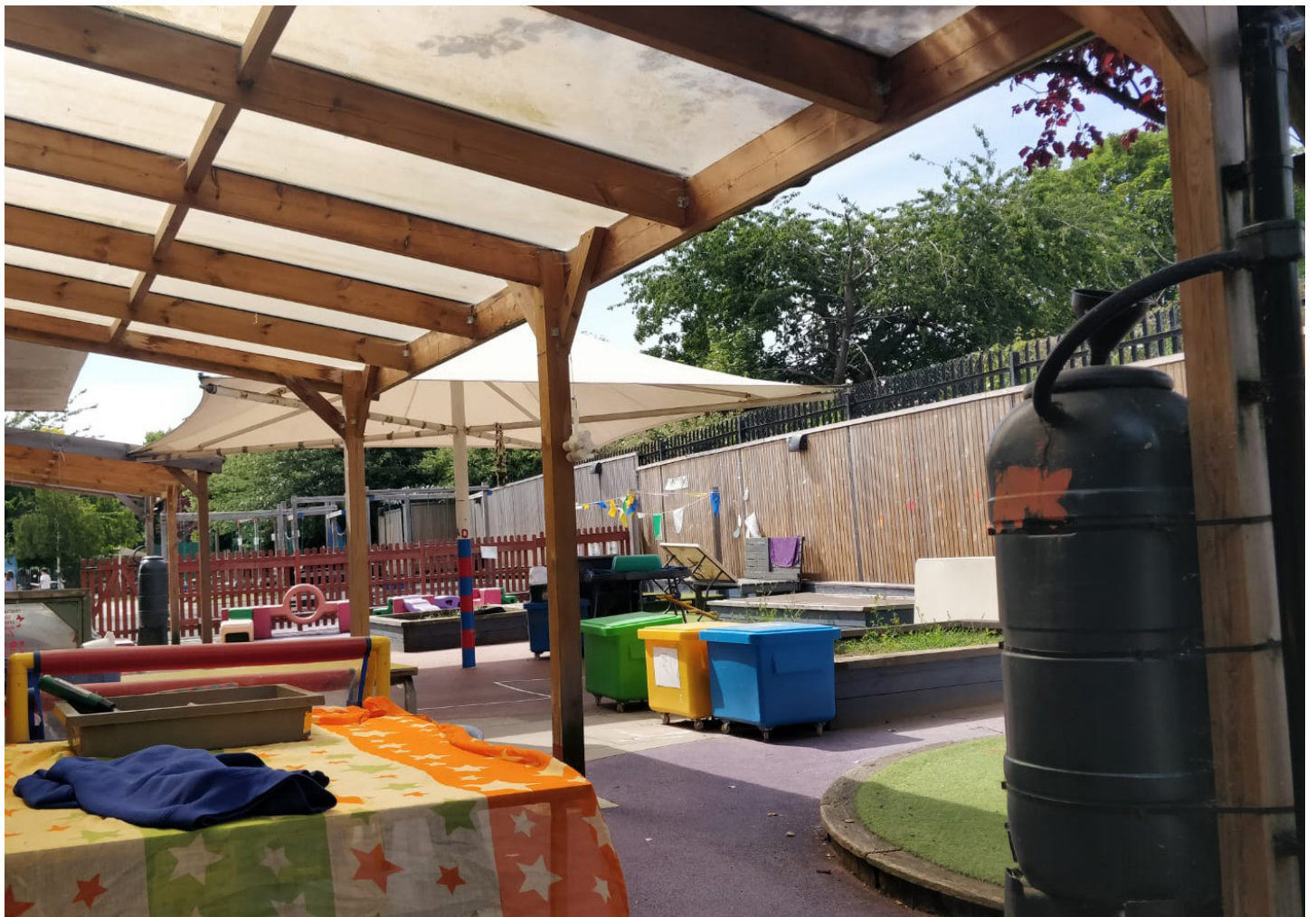
A water-harvesting system at Southern Road Primary School
