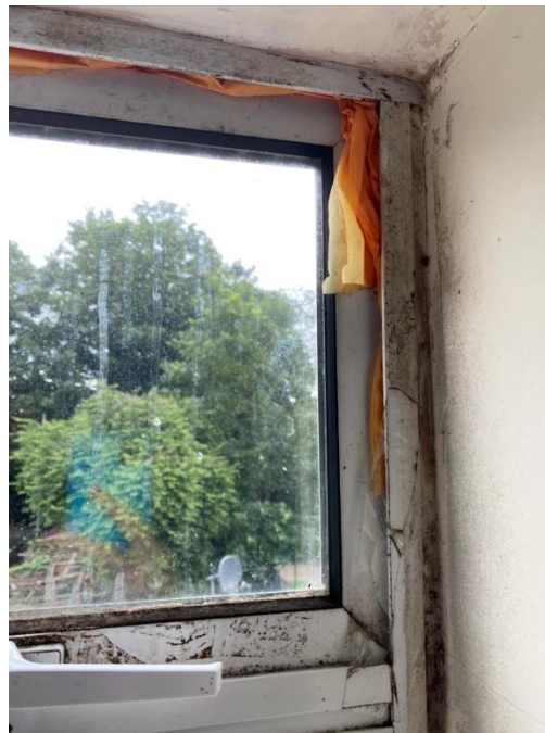
Left photo: shows dampness and mould growth with a large hole in the rear wall of the bathroom.
