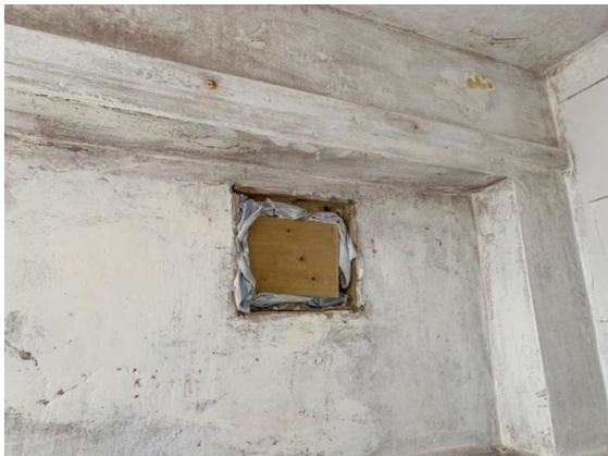
Left photo: shows dampness and mould growth with a large hole in the rear wall of the bathroom.
