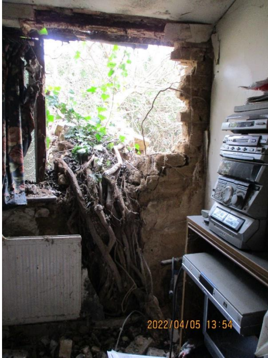
Photos above show the hole in the wall from the tree, exposing the tenants to the elements and making the structure unsafe and unstable.
