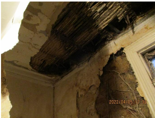
Photos above show the hole in the wall from the tree, exposing the tenants to the elements and making the structure unsafe and unstable.
