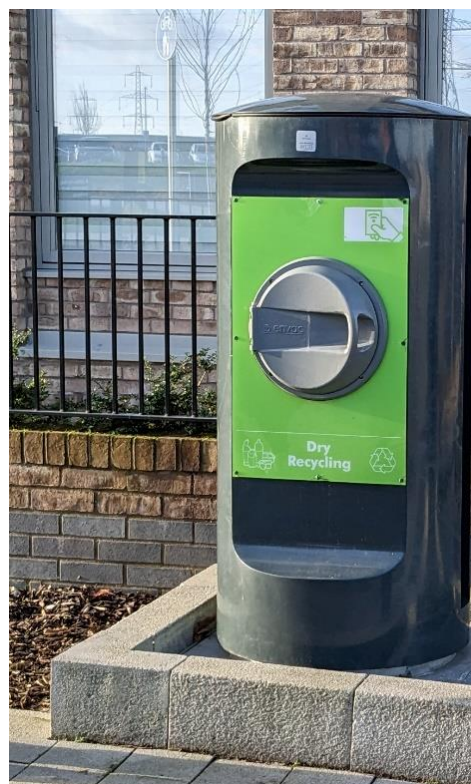
Figure 1: Example of an on street disposal inlet
