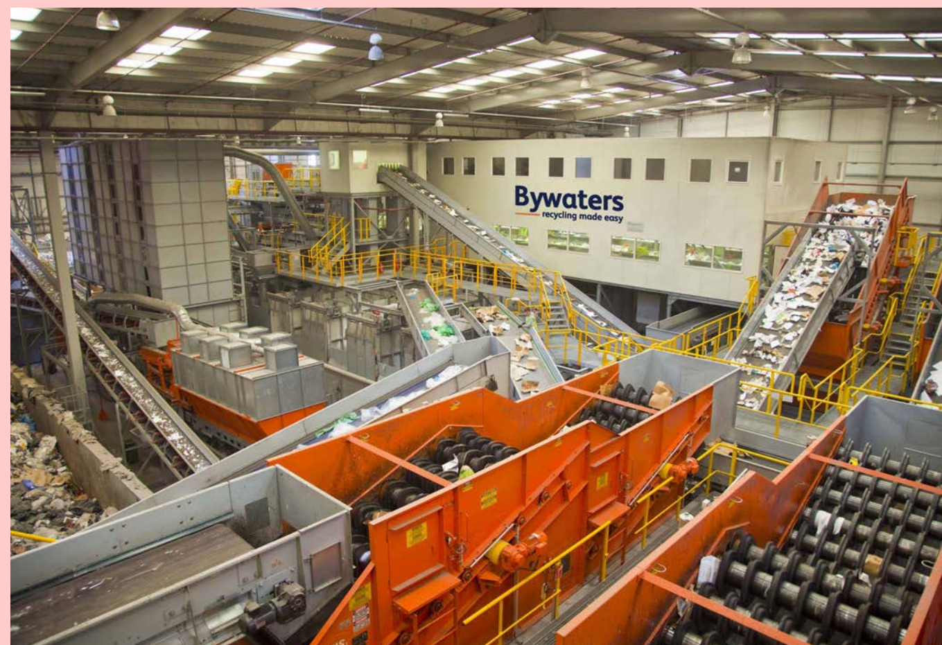
Fig. 27 + 28: Aerial image of the Bywaters recycling facility and internal image of the facility.
