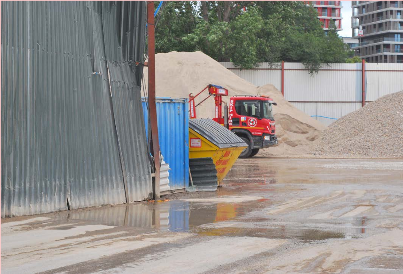
Fig. 29 + 30: RMS: Concrete Recycling Facility.
