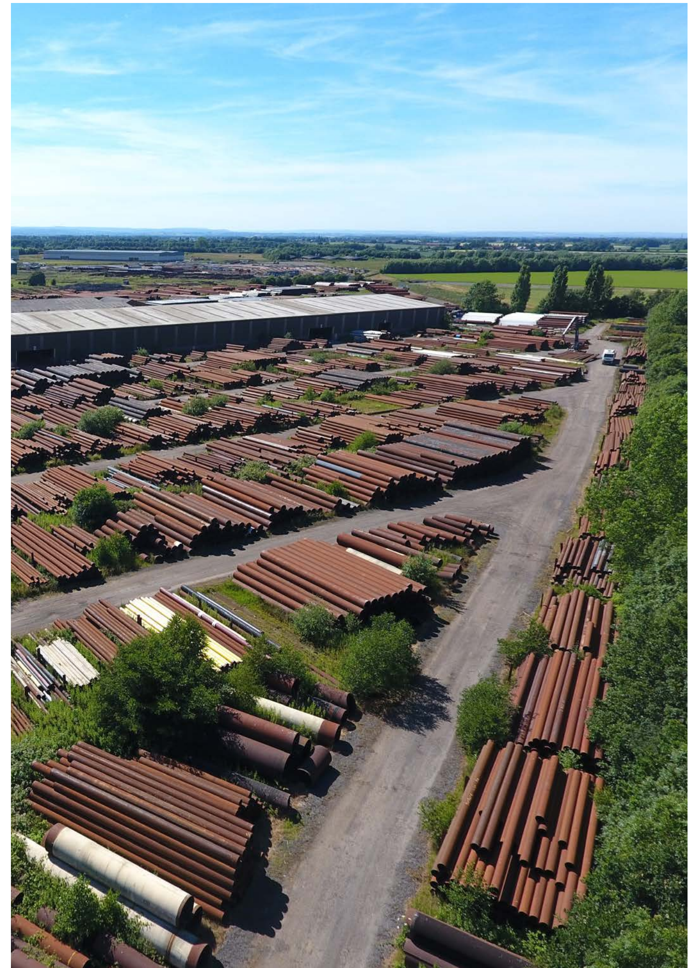
Fig. 3: Aerial shot of steel pipework stock at Cleveland Steel.
