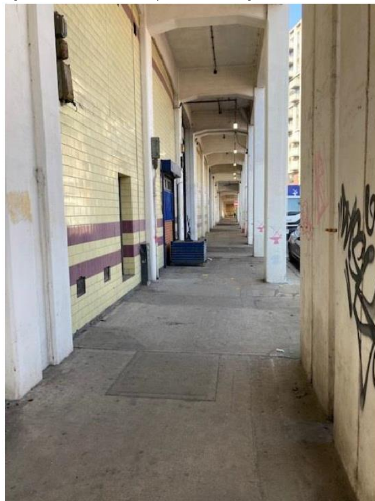
Figure 10: Silvertown Way arches looking North West
