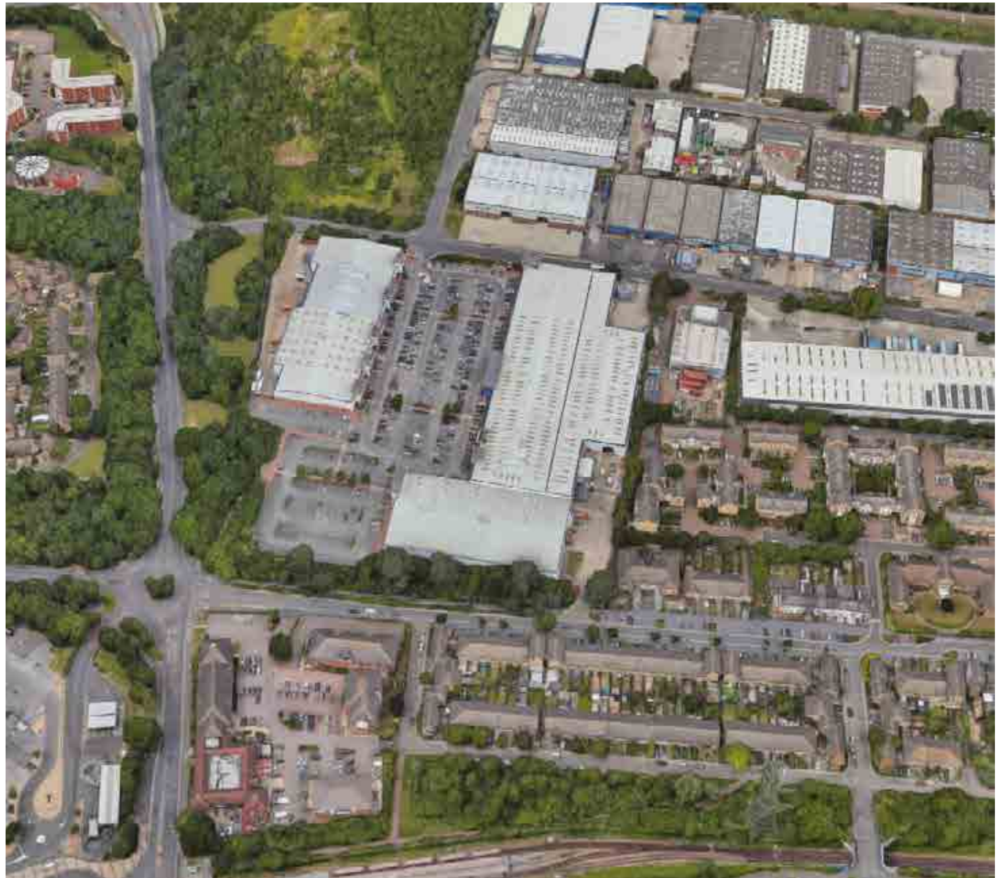
Fig 35 Alpine Way industrial site view
