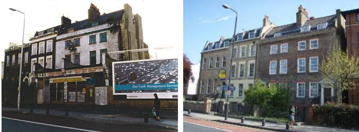
58, 56 and 54 Romford Road before and after restoration
