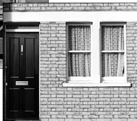
*The original style of window opening and surround must be kept and, where a new window is installed, such as in this annexe, should replicate an original design.*
