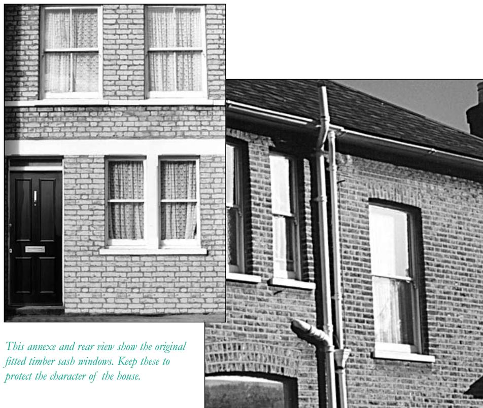
*This annexe and rear view show the original fitted timber sash windows. Keep these to protect the character of the house.*
