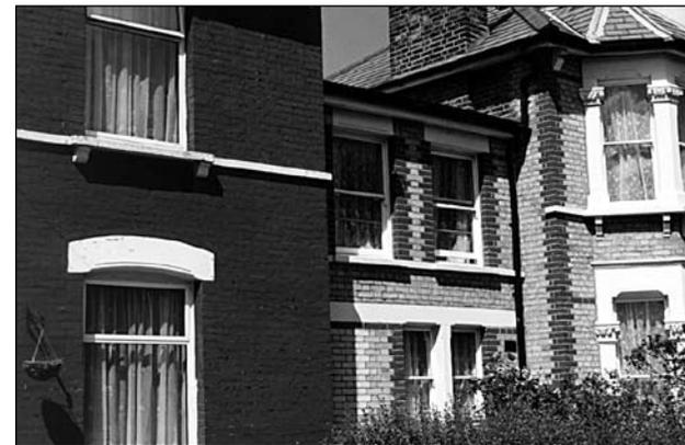
*Painting of the house on the left in the above picture has hidden the lively colour contrast of the original brickwork as shown on the house next door.*
