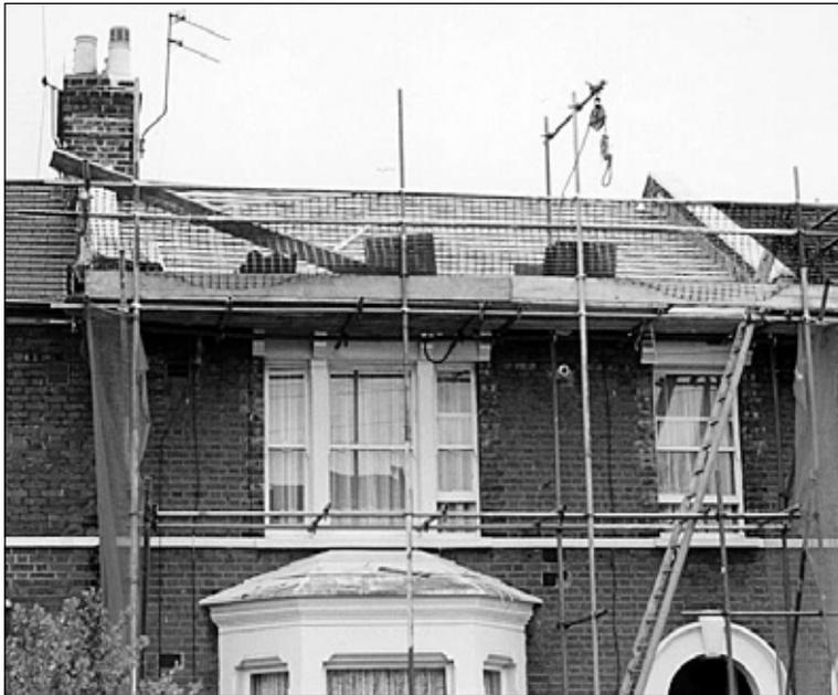
*Work in progress. If a roof is being re-covered only natural or artificial slate is acceptable.*
