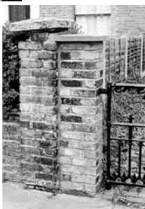
▶ Right: Jointly owned piers were provided at boundaries. Hang gates from these. Build new walls to the height of adjoining original walls to produce a neat unified streetscene.
