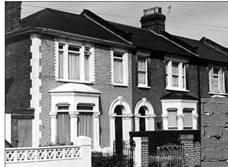
*The unity of this terrace has been ruined by the painting of the brickwork on the end house. Painting can harm brickwork and require costly maintenance (see detail). It should be removed rather than repainted.*
