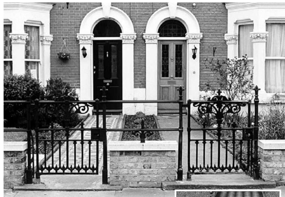
▲ Above: A well thought out joint scheme renewing gates and walls. Note gates are hung from posts as they would have been originally.
