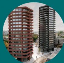
New housing blocks
